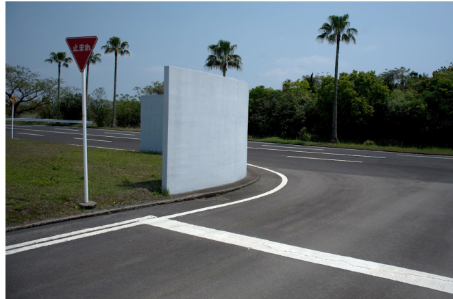
Blind corner. Course 1 (#34,35) / Course 2 (#23,24)
